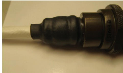
Figure 73: Shrinking tubing over backshell
