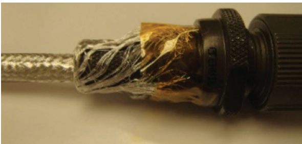
Figure 38: Returning braid to connector
